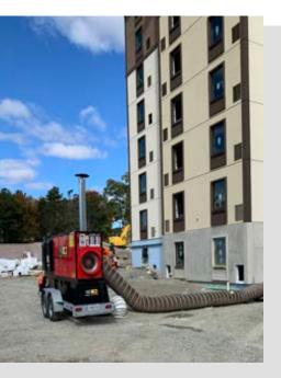
**Customized Rental Heating –** Placed outside the building, and fed through temporary ducting, two trailer-mounted 1 million btu indirect fired heaters were delivered just as it turned cold. With a large footprint across the building, each unit heated a separate floor, with air delivered evenly across the floor using temporary poly-tubing. As the contractor completed drywall, taping and painting, the heat was directed to another floor, simply moving the temporary ducting.
